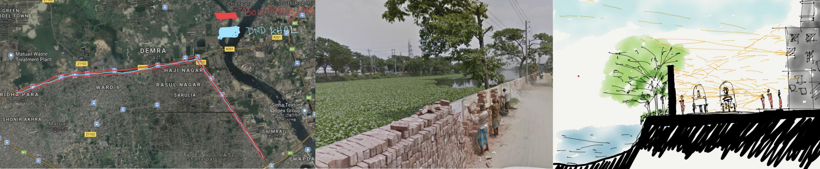
A boundary wall approximately 7.2 kilometers long separates the canal from the surrounding communities.
