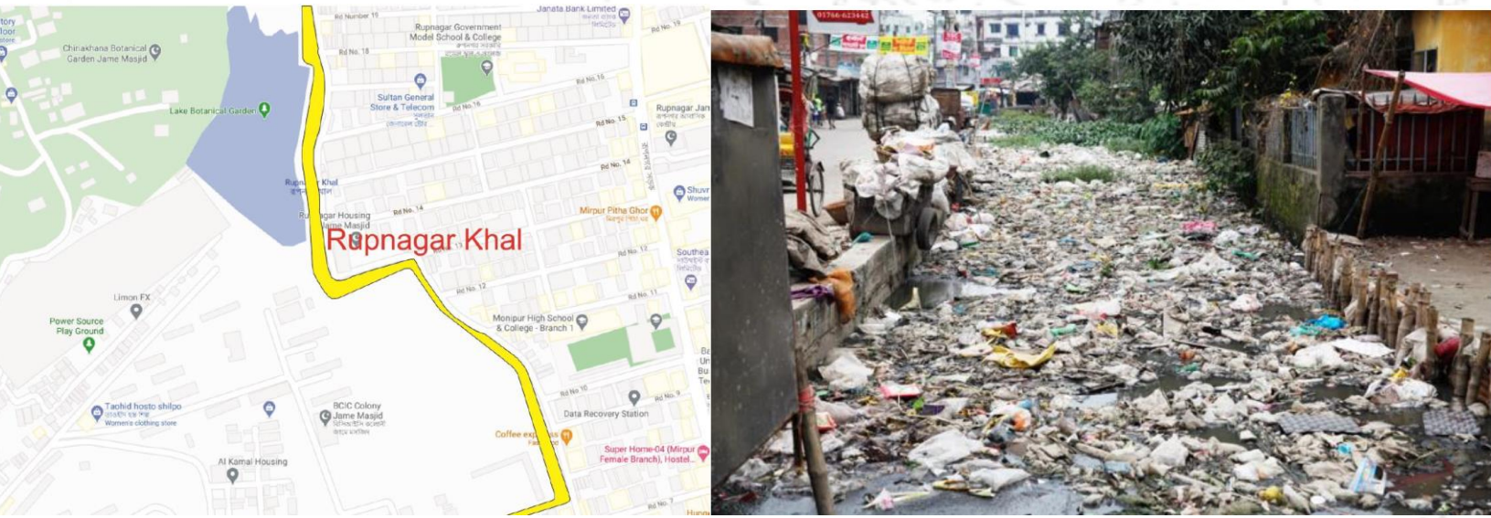
Rupnagar has an inadequate drainage system. Most drains are blocked with waste.
