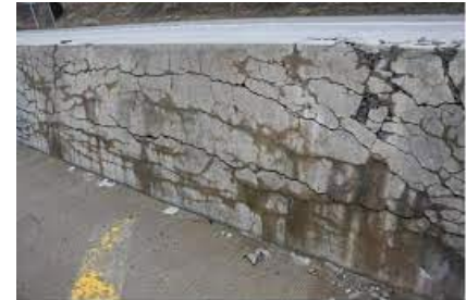
Fig. 1.1-1 Typical deterioration in concrete barrier
