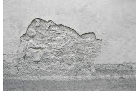
Fig. 1.1-1 Typical deterioration in concrete barrier
